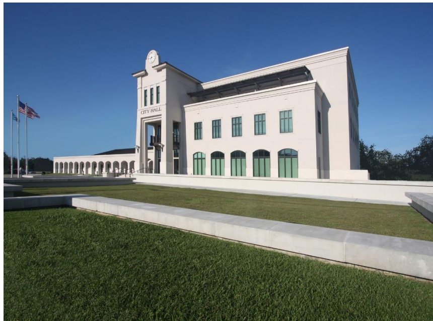
Figure 5: D’Iberville City Hall, a TOMAS 3 building. The building includes historic elements, such as a cornice and arched windows, and modern elements, such as an asymmetric design. Photo by Patricia W. Hughes courtesy of Eley Guild Hardy.
