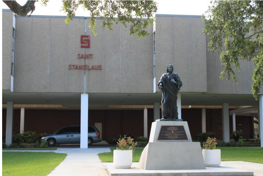
Figure 6: Saint Stanislaus College, in Bay St. Louis, a TOMAS 4 building. Photograph by author.
